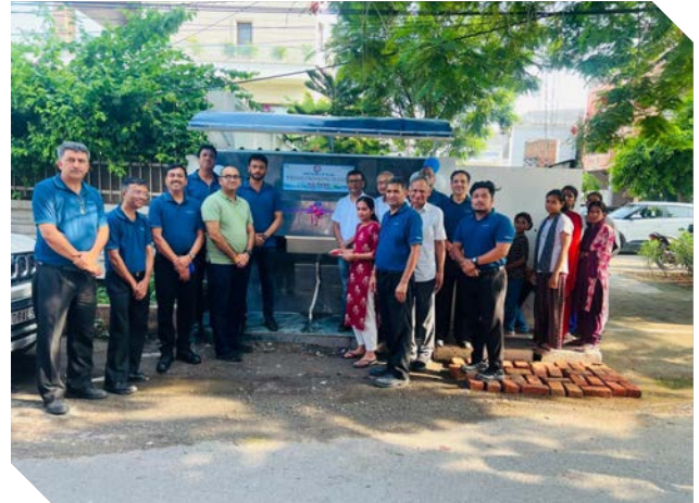
► Civil works and installation of a drinking water facility at Rotary Saheli Centre, Rudrapur
